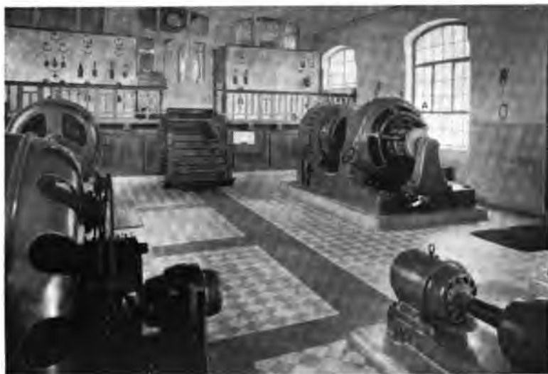
FIG. 149.—Generating plant at Nauen: A. alternator; B. generator.
